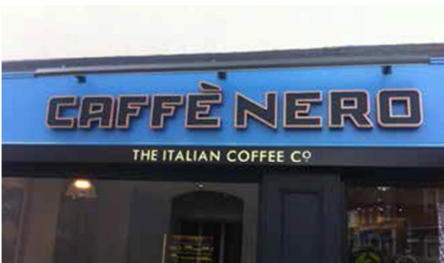
Contemporary style fascia
