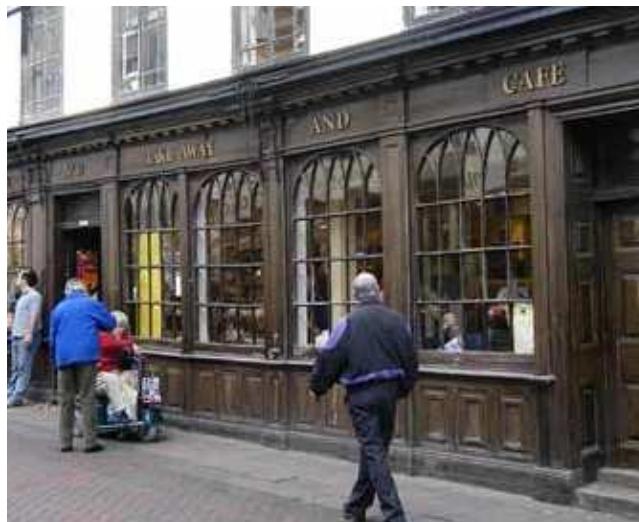
Traditional timber stall riser
