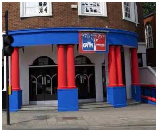
Inappropriate use of visually dominant colours
